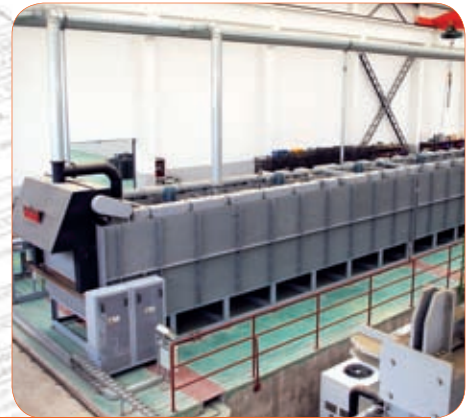
▶ Aichelin heat treatment line (100 m. long)
